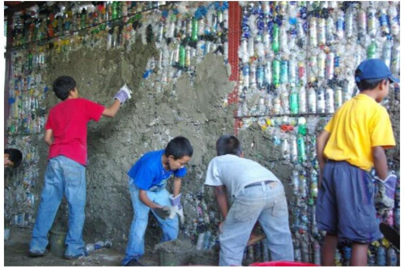
Applying cement to the inside of the building...
