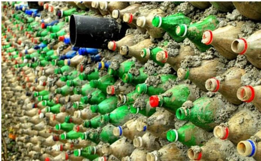
A bit more cement will be applied and smoothed out.
