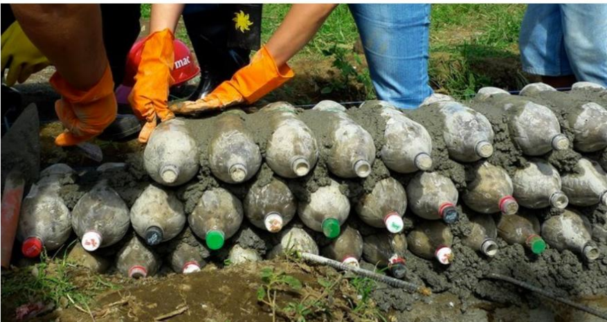
The building process begins. Pic: micealiling.com
