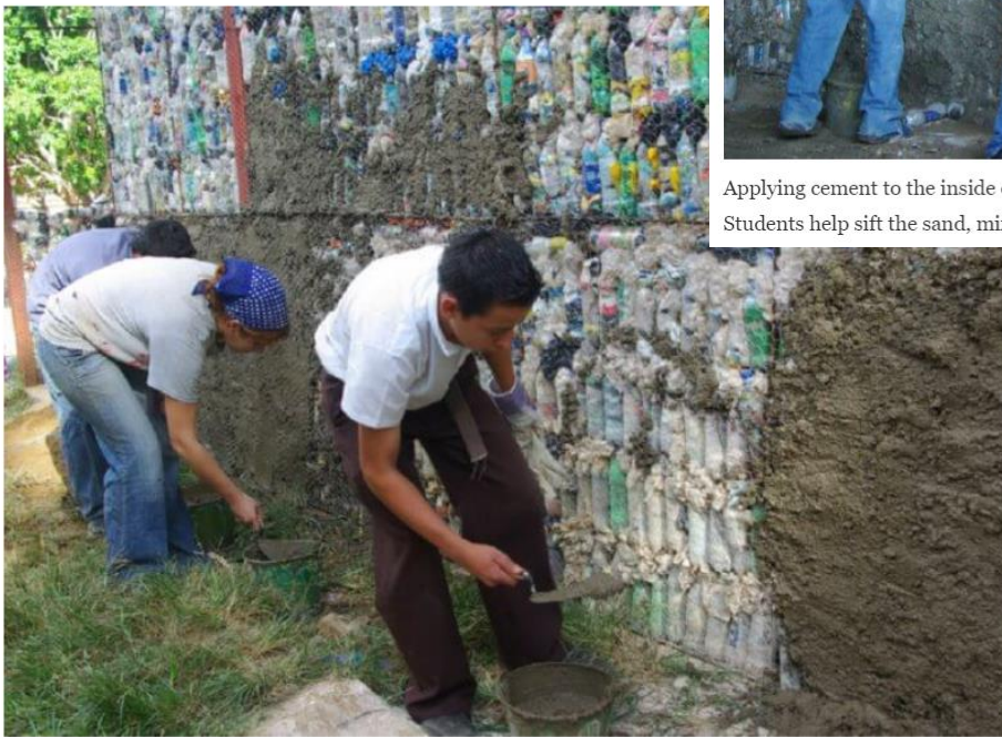
And on the outside... Three layers of cement are applied. www.flickr.com
