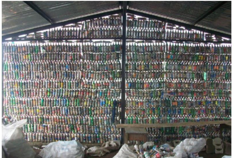
This school used metal frames instead of cement posts. hugitforward.com
