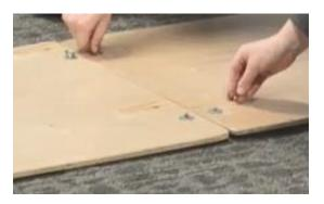
Use 6 connectors and 4 carriage bolts and washer and wingnuts per connector.
